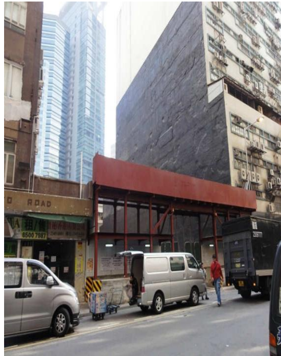
Current Situation (Demolition completed)
