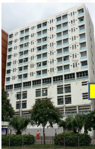
Original building on the land before demolition
