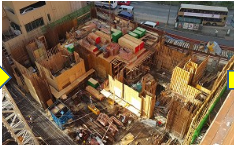
Site under construction
