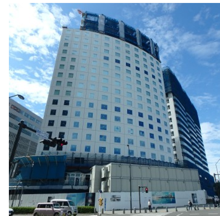
Current construction progress
