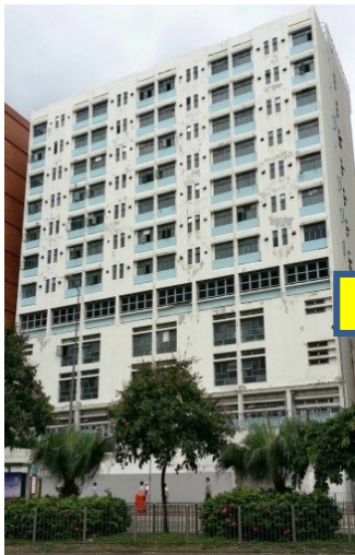
Original building on the land before demolition
