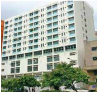
1. Original building on the land before demolition
