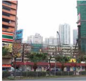
2. Site after demolition of original building
