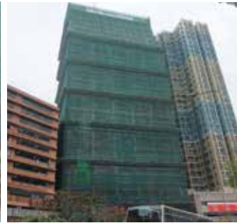
3. Site under construction
