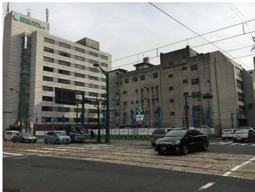
Existing site after demolition of original building
