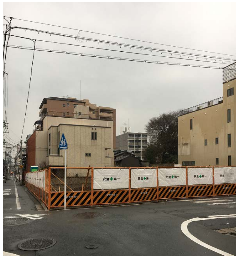
Existing site after demolition of original building
