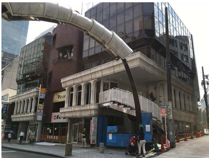
Original building at the site before demolition
