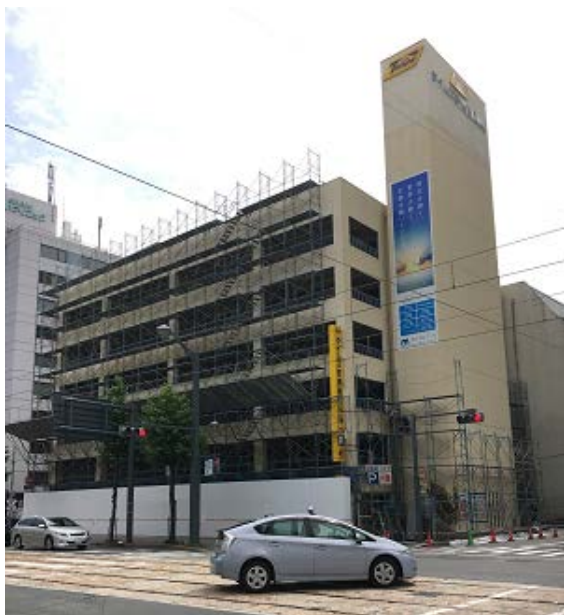
Original building at the site before demolition
