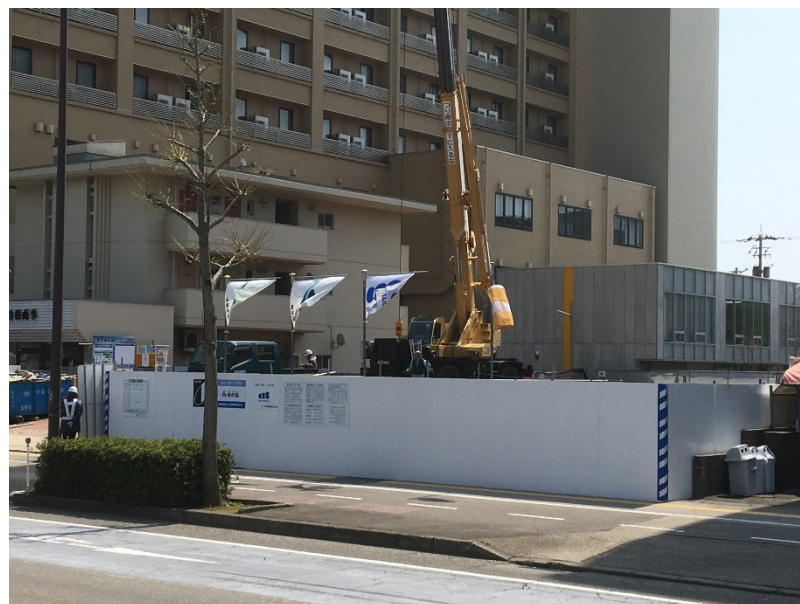
Existing site undergoing construction
