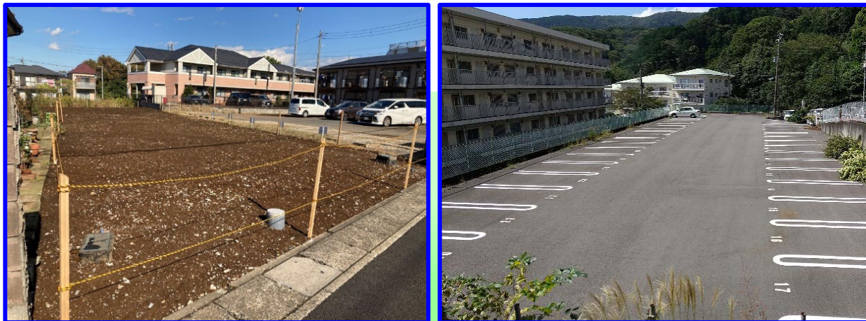
Pictures of the two group home construction sites:
