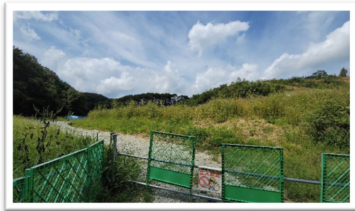
Site of Otawara Solar Power Plant
